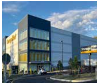
Storage Mart has recently completed construction on Salem Lane.
