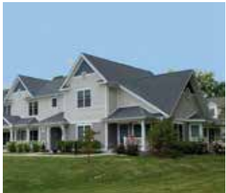
Lascana housing development includes 46 units including 36 units of affordable housing.
